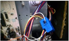
WARNING: If the SCT013 current probe jaws are not completely closed -- then the current measurement by the SYSTEM will be adversely affected. The SYSTEM will not operator and/or will operate inconsistently. Clamping the SCT013 current probe around both wires WILL give you a zero reading and the MCerberus® unit will not operate correctly.
